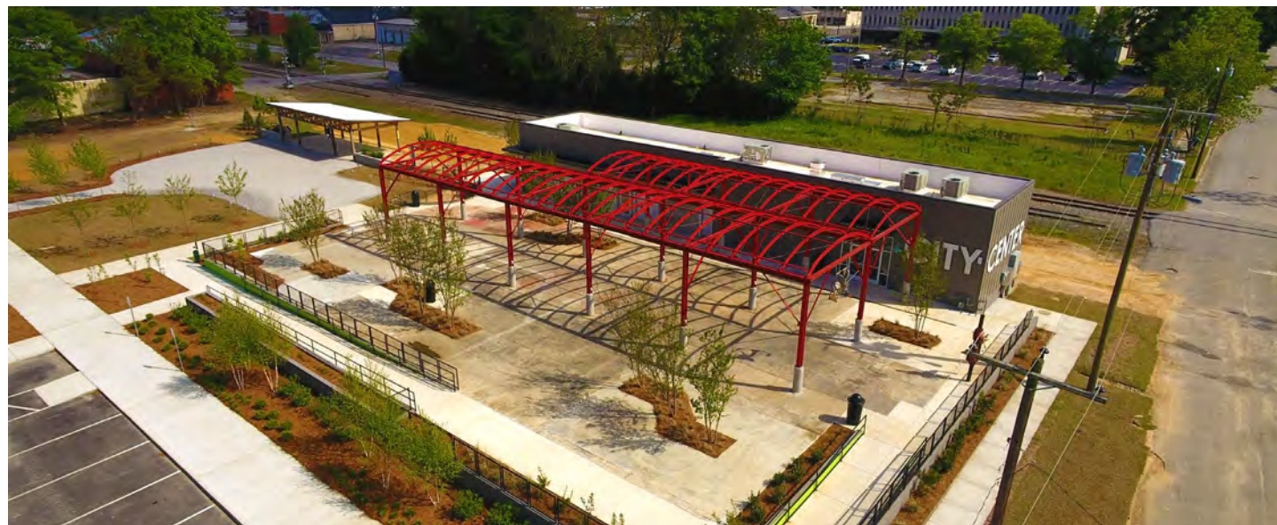
The Florence City Center Market and Kitchen includes a space with an awning for farmers market vendors. Photo sourced from the Florence Downtown website.
